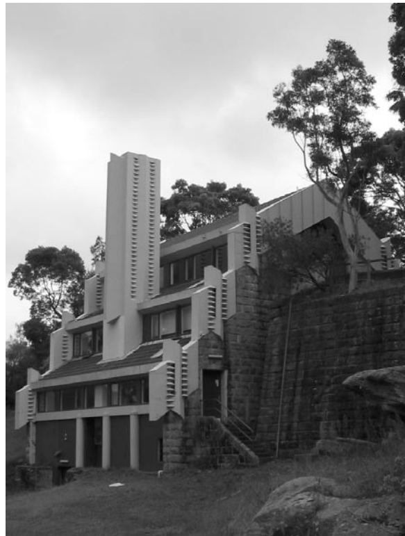
Willoughby Incinerator photographed in 2005 showing the truncated chimney stack. The top decorative element was removed in 1954.
